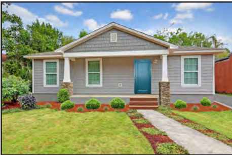
Category 1 - Under $160,000 Pensacola Habitat for Humanity 816 West Belmont Street, Pensacola West Side Garden District
