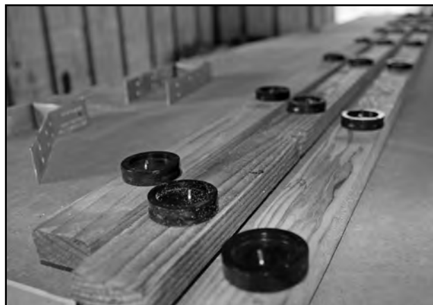
Small, plastic risers on the roof battens allow for improved air flow and water drainage.
